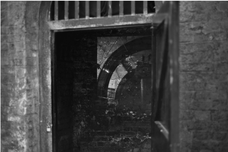
Figure 4.7 View into coal hole, with projection of turbines at Kew Bridge Steam Museum 3
