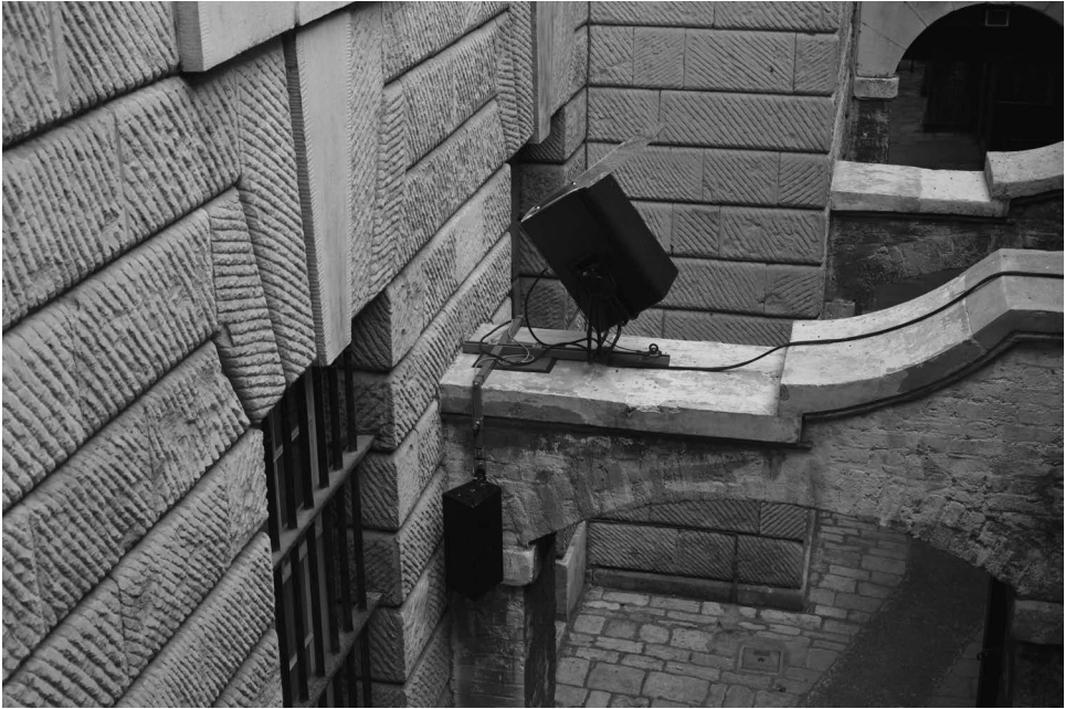
Figure 4.4 View from mezzanine level of part of the system of speakers, Somerset House light wells Source: Bill Fontana, photo by Claire Reddleman
